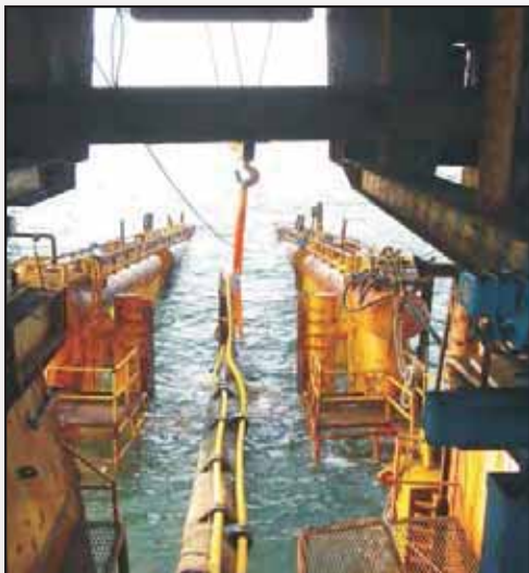
DDWFDP – Pipeline laying by pipe lay barge
