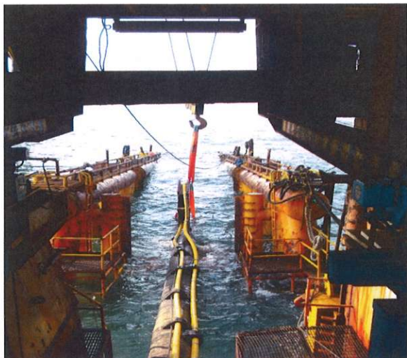
DDW FDP – Pipeline laying by pipe lay barge
