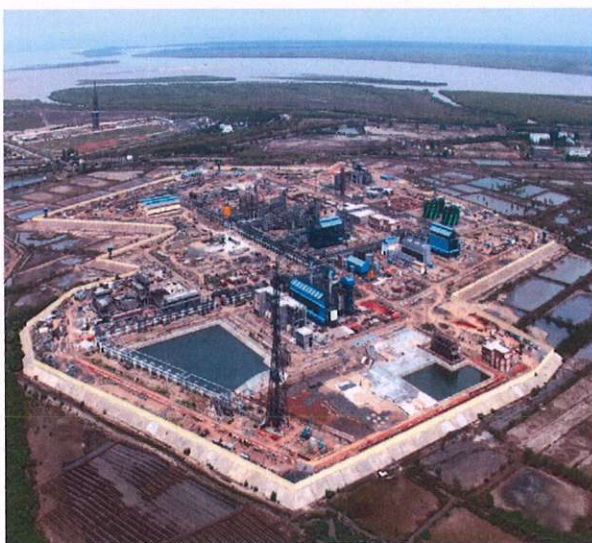
DDWFDP – Aerial view of OGT
