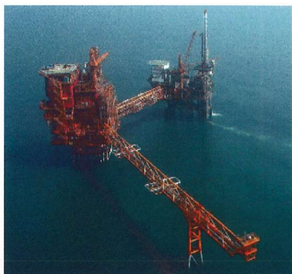
DDWFDP – Aerial view of WHP & PLQP
